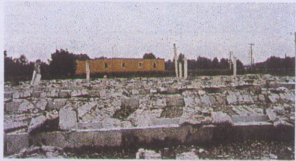
Photograph 3 Building Type C
