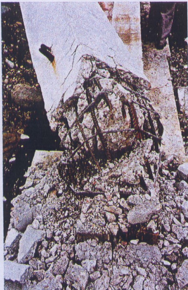
Photograph 1 Column in Building Type A
