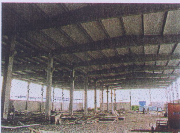
Photograph 5 An undamaged precast concrete structure
